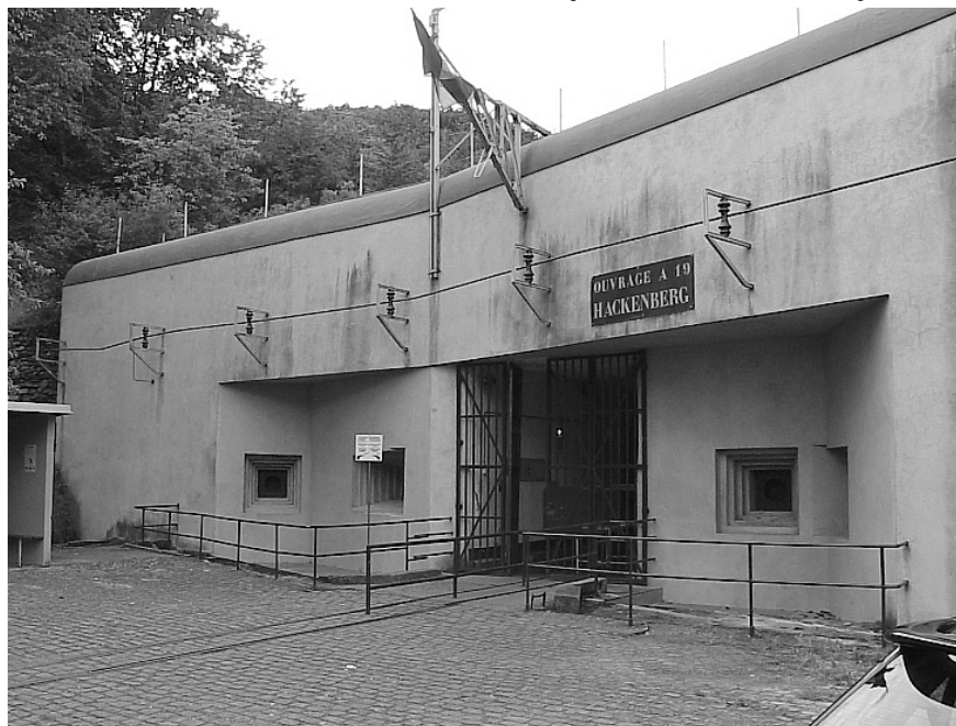
Hackenberg - Munitions Entrance Photo Dan McKenzie
